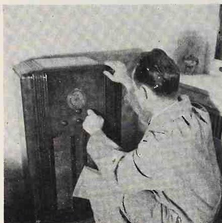
Carefully re-install set, tighten knobs.
