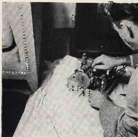
Repair slipping dial drive mechanisms.
