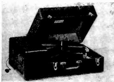
Model SRC-4 portable record player, 4 tubes, ac, handling 10" and 12" discs with cover open or closed. Crystal pickup, 6 1/2 watts undistorted output, 78 RPM constant speed synchronous motor with 9" turntable, 6" dynamic speaker. Controls for volume and variable tone. Plywood construction covered with simulated alligator skin leather, "luggage" style. (Model SRC-4 was formerly tagged SRC-2). Musitron Co., 223 W. Erie St., Chicago 10, Ill.—RADIO & Television RETAILING
