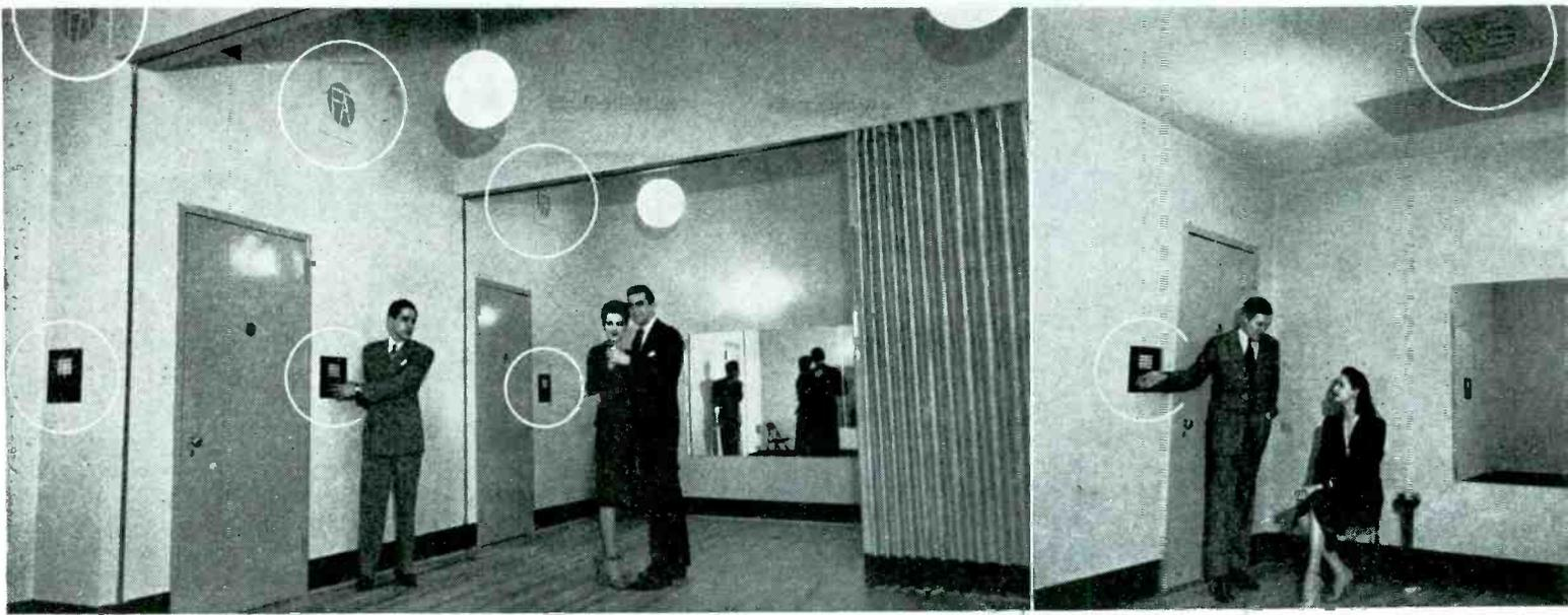
While overhead location is preferred, wall installations of the 12" General Electric cone PM speakers are also used. At left, Buddy Eisen, who sold the system, checks out the selector box associated with the speaker directly above. Each of the three studio sections has its own setup.
