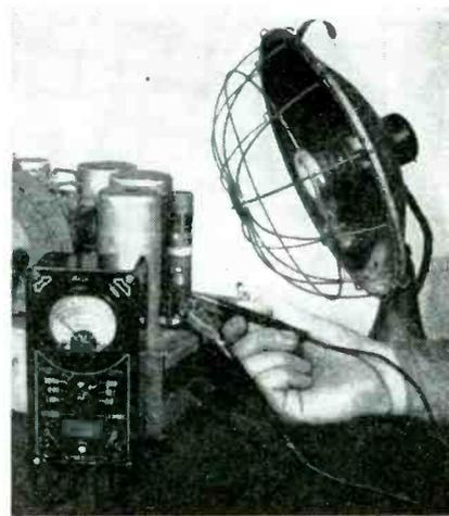
Applying radiant heat to "force" troubles.
