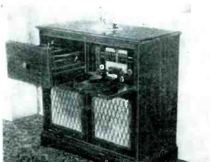
Model G-722 radio-phonograph console, standard broadcast plus shortwave. Push-button tuning, 10" speaker, all-directional built-in aerial. Newly designed fool-proof automatic disc changer playing 10" and 12" records intermixed with automatic shut-off. Extra storage space for albums. Cabinet of rare wood and mahogany veneers. Templetone Radio Mfg. Corp., New London, Conn.—RADIO & Television RETAILING
