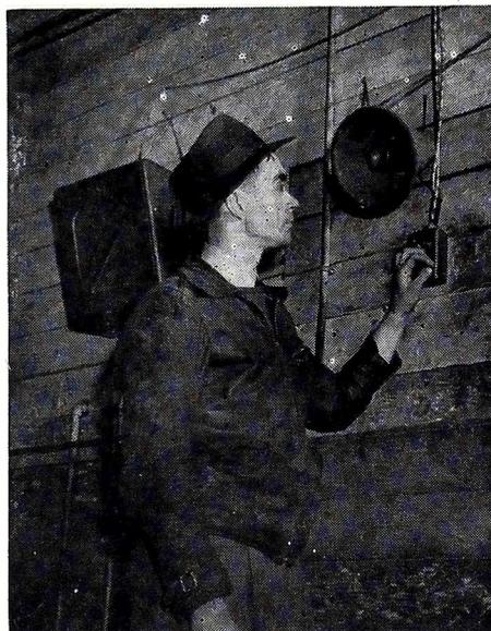
▲ Wooden baffle speaker at left, part of paging system, is possible here because of low dust level in scrap room. ▼ Below, one of two centralized amplifier banks in the laboratory.
