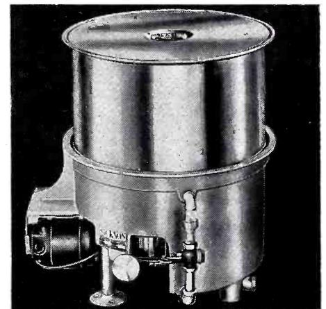
own motor-operated centrifugal pump, used to recirculate the water, drawing it through the bottom from the fine strainer which collects refuse.  $2\frac{1}{2}$  gallons of water required to fill wash reservoir. Two baskets are furnished, one for dishes, one for glasses and silverware. Optional equipment includes electric immersion heater and thermostat control. The Jackson Dishwasher Co., 3703 W. 93 St., Cleveland 5, O.—RADIO & Television RETAILING
