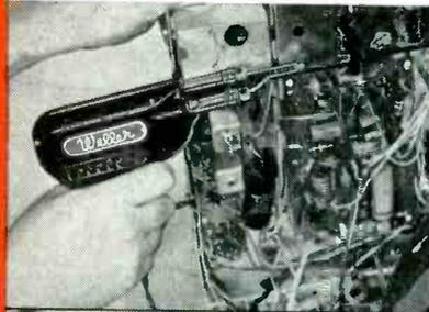
**2 REACHES COMPONENTS THROUGH CHASSIS CUT-OUTS.** Weller Guns, with their long, thin electrodes, reach recessed tube sockets and connections through small chassis cut-outs. Pre-focused twin spotlights light up this hard-to-get-at work.
