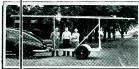
The new Price Tenna-Trailer will put you way out front of your competition. It enables you to quickly raise a 51 foot mast. One man can set the versatile unit in position, crank up telescoping mast, rotate for best signal — all in a matter of minutes. You'll be thrilled with its ingenious, sturdy construction!
