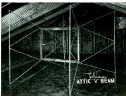
The array is extremely light and entirely self supporting. It may be suspended or rested on flooring, beams, rafters. The Attic "V" Beam is said to make outdoor installations unnecessary in nearly all locations within a radius of 30 miles from TV stations without sacrificing picture quality and overall performance. Telrex, Inc., Asbury Park, N. J.—RADIO & TELEVISION RETAILING.
