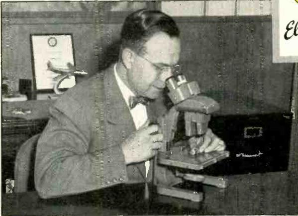
● A General Electric executive micro-inspects a tube structure for proper assembly.
