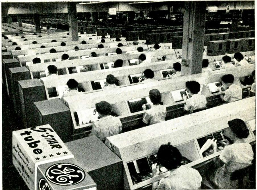
**BUILT UNDER GLASS IN LINT-FREE FACTORY!** No dust, lint, moisture get in 5-Star Tubes to affect performance. Rubber finger cots keep workers' hands from touching mounts. Pre-cleaned parts are delivered to the assembly area in sealed containers.
