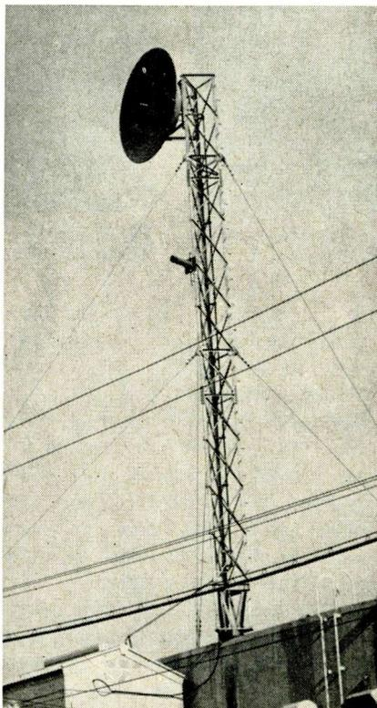
Fig. 7—450 mc helical and 6000 mc parabolic antennas mounted on the same mast.
