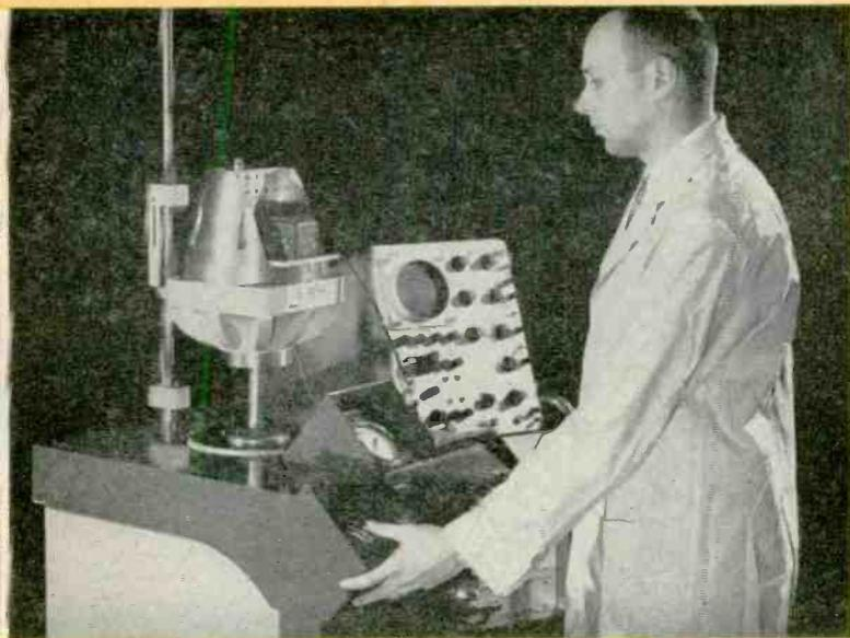
Avco shock test machine for electronic components tests a relay with a 30 g, 11 millisecond half-sine shock. It can test up to 3000 g. There is no superstructure, and the machine relies on air pressure to propel it down during test.
