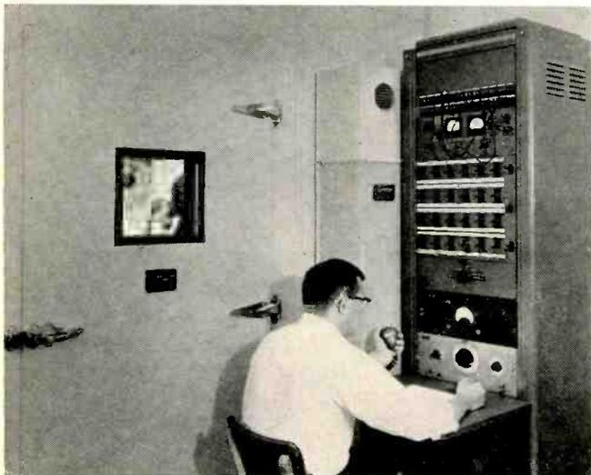
This Shure Brothers sound room is where the company is developing special-purpose mikes that can be used in noisy environments. For example, inside the 6 x 6' insulated room, engineers can duplicate the roar of a jet engine at 500 feet, unbearable to the human ear except for a few minutes.
