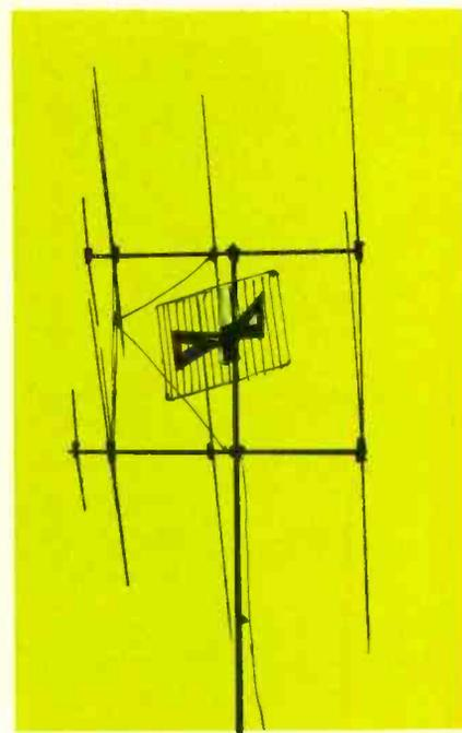
UHF antennas mounted on the mast in this position can and usually will give erratic reception.
