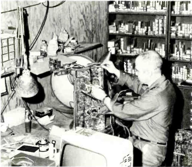
Service technician makes voltage tests on printed circuit board of TV chassis.
