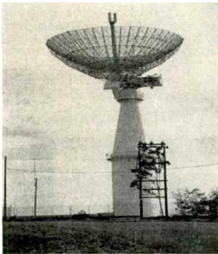
Fig. 1—84-foot diameter "dish" on its 90 foot tower used to bounce radio signal from the planet Venus back to earth. Signal took about 5 minutes for round trip.
