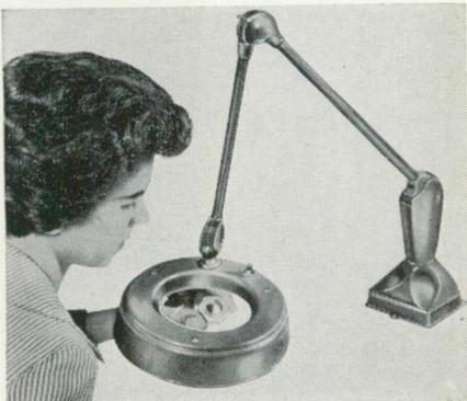
diameter, focal length 13", power, 3 diopters, for distortion free magnification; and 26" swinging arm. Available in four models. Acme Lite Products Co., Congers, N. Y.
