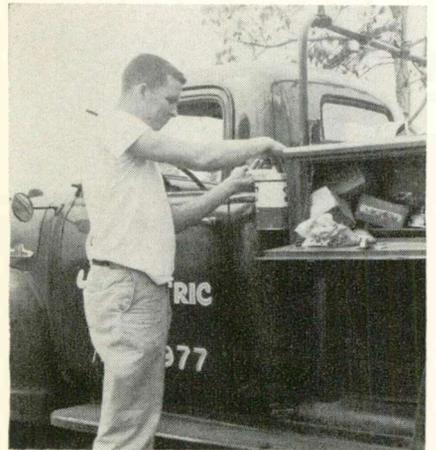
Fig. 4—Vehicle-mounted waterless hand cleaner helps techs maintain clean appearance without using customer's washroom.
