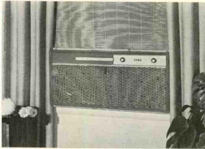
Fig. 1—Typical completed double-window home air conditioner installation showing inside flush-mounted Remington conditioner unit.
