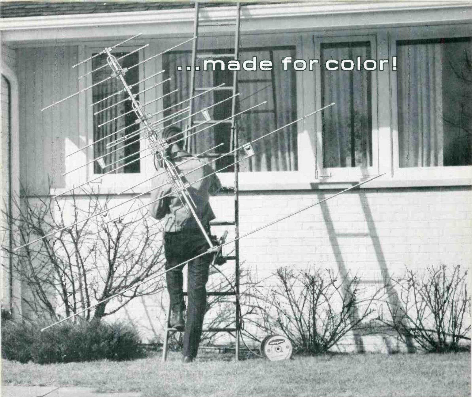
**Directivity**—Equally important for superior color pictures is freedom from interference and ghosts. Therefore, an antenna with sharp directivity and good signal-to-noise characteristics is necessary. Extraneous signals picked up at the back and sides produce objectionable noise and ghosts in black and white reception . . . frequently ruin color reception.
