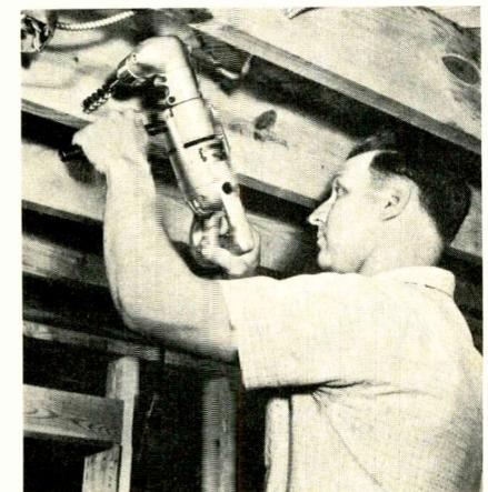
Sound system installers find this drill made by Black & Decker particularly valuable where cables must be run through joists.
