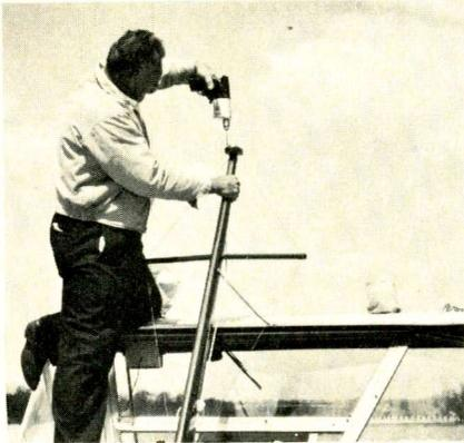
Drilling the mast of a boat for an antenna with a battery-powered drill. It is strongly urged that this type shoe not be worn on boats if you ever want to do more work for the owner.
