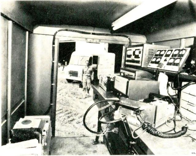
Inside view of a truck equipped to test and repair two-way radios.
