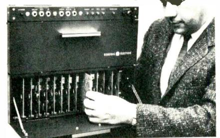
Dial-paging terminal equipment made by G-E for PBX-equipped buildings. Equipment allows direct voice message from any plant telephone to radio-equipped men on the move.
