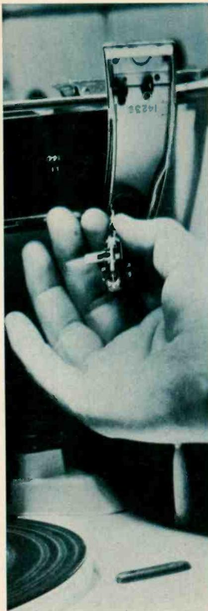
Replacing cartridge in portable stereo record changer.
