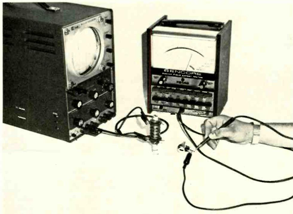
Fig. 14—An electronic technician is shown measuring the resistance of a potentiometer to determine the ac resistance of the coil.
