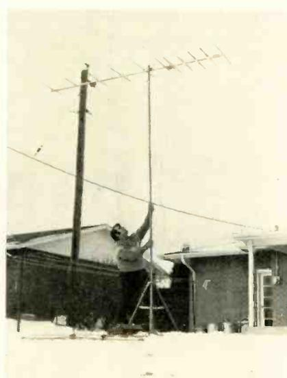
Rough orientation, once the test antenna is up, is the first step in determining the direction for best signal reception.
