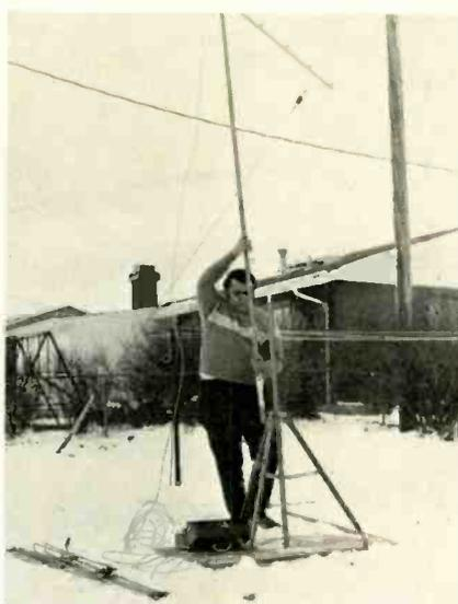
Up goes the top section as Joe Barno prepares to test signal strength with an antenna cut to Channel 9. The home owner at this location has had a weak signal problem on this channel.
