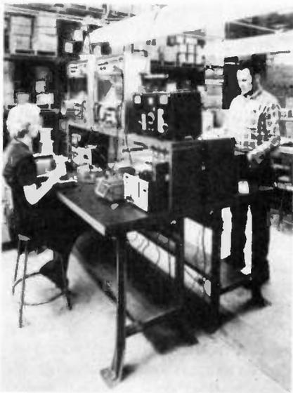
over steel top are available in 10 sizes ranging from 48 in. wide, 28 in. deep, and 30¼ in. high, to 72 in. x 34 in. x 34¼ in. Standard accessories include: stringers, shelves, back and end stops, risers, electrical outlet strips, case and drawers with one tray and bench drawer mounting kits.
