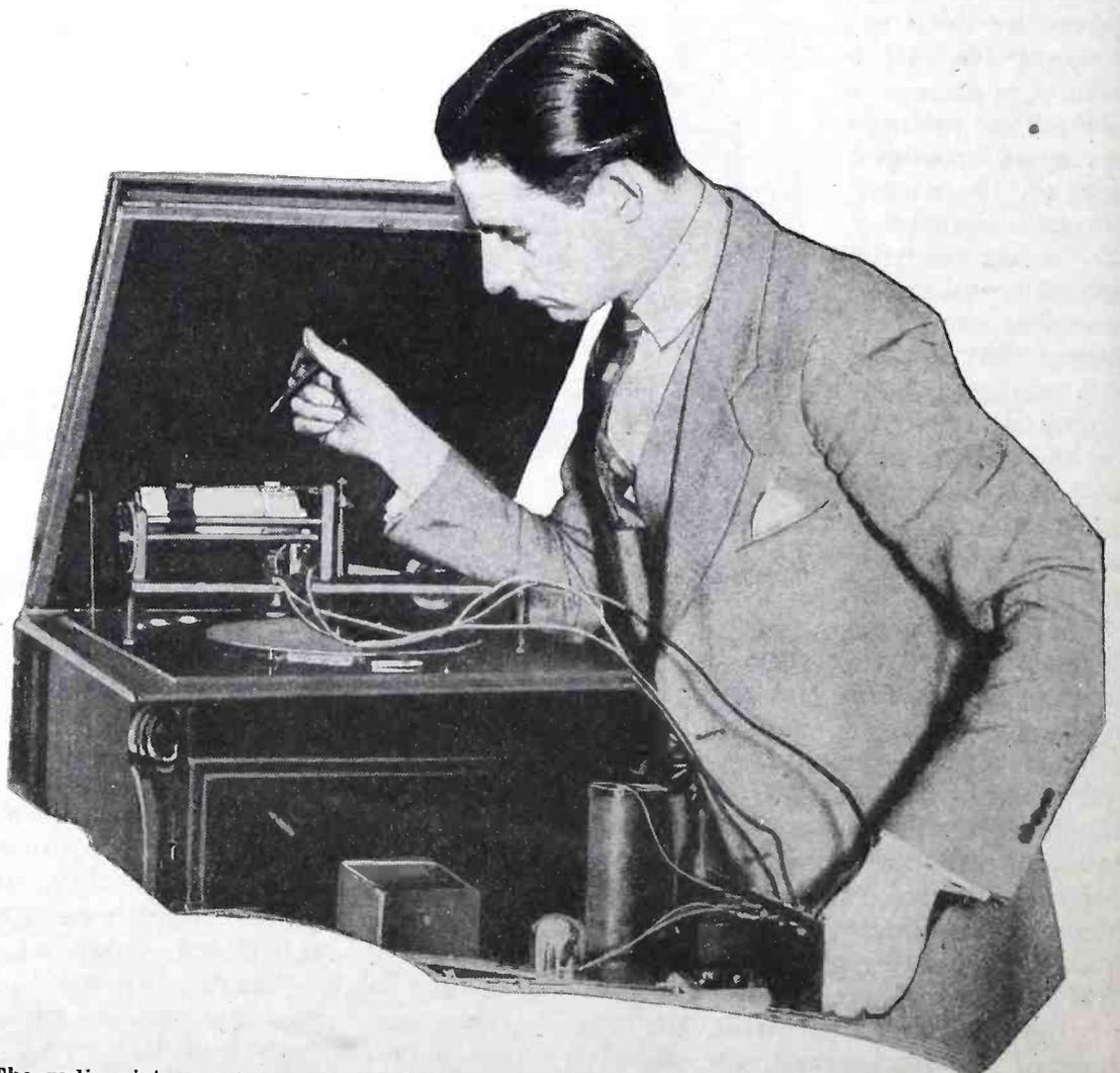
The radio picture set receiving a photograph with the aid of a victrola motor as the driving device. Experiments are being conducted daily with radio picture sets such as described in this article.
