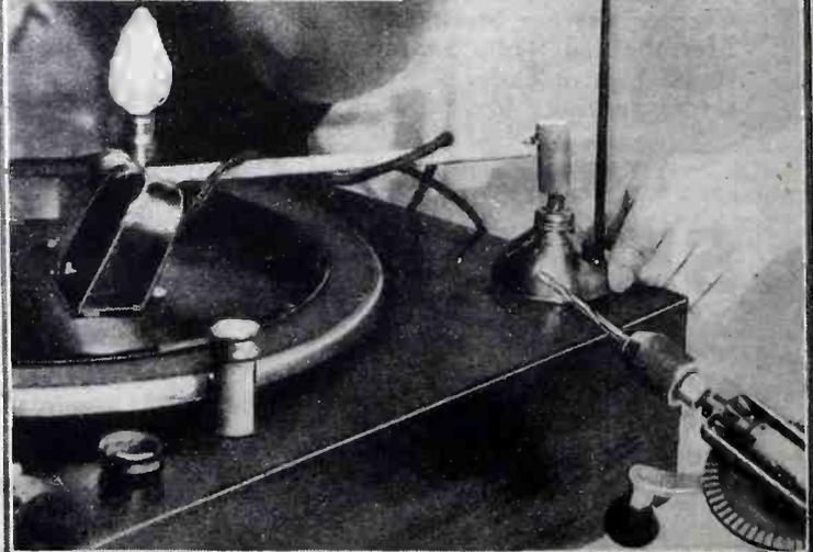
One length of dowel stick, one-quarter inch in diameter and about a foot long; two smaller pieces of dowel, one-half or five-eighth inch in diameter and each two inches long; a small brass hinge, not over one-quarter inch wide; and a small oil can.
