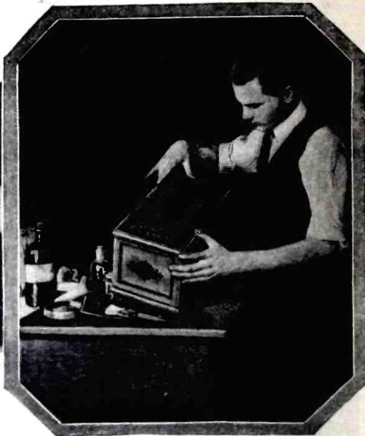
Left, rubbing down first coat of varnish with powdered pumice stone and rubbing oil; right, radio cabinet finished in antique after it was completed.
