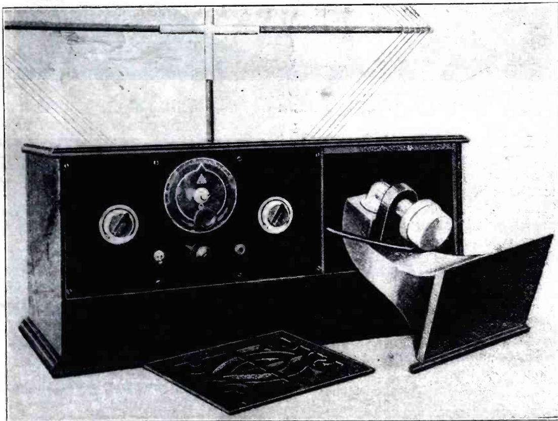
A front view of the set with the loud speaker unit and horn removed. The dial used on the shaft of the variable condenser is preferably of the vernier type in order to provide micrometer control.
