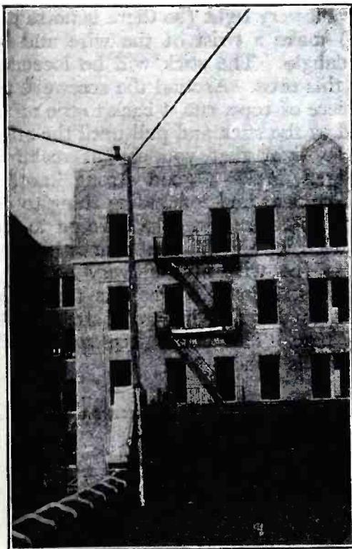
Fig. 5, showing a view of one of the poles. The guy wires are difficult to see, due to the similar background. Note the height of the pole, and how the antenna is continued right through the insulator.
