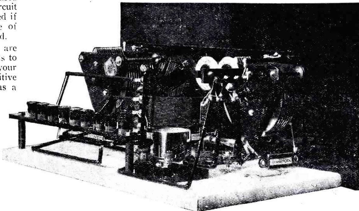
Fig. 12. A perspective of the completed frequency changer. The grid leak and condenser are supported by the tube socket and the wiring to it.
