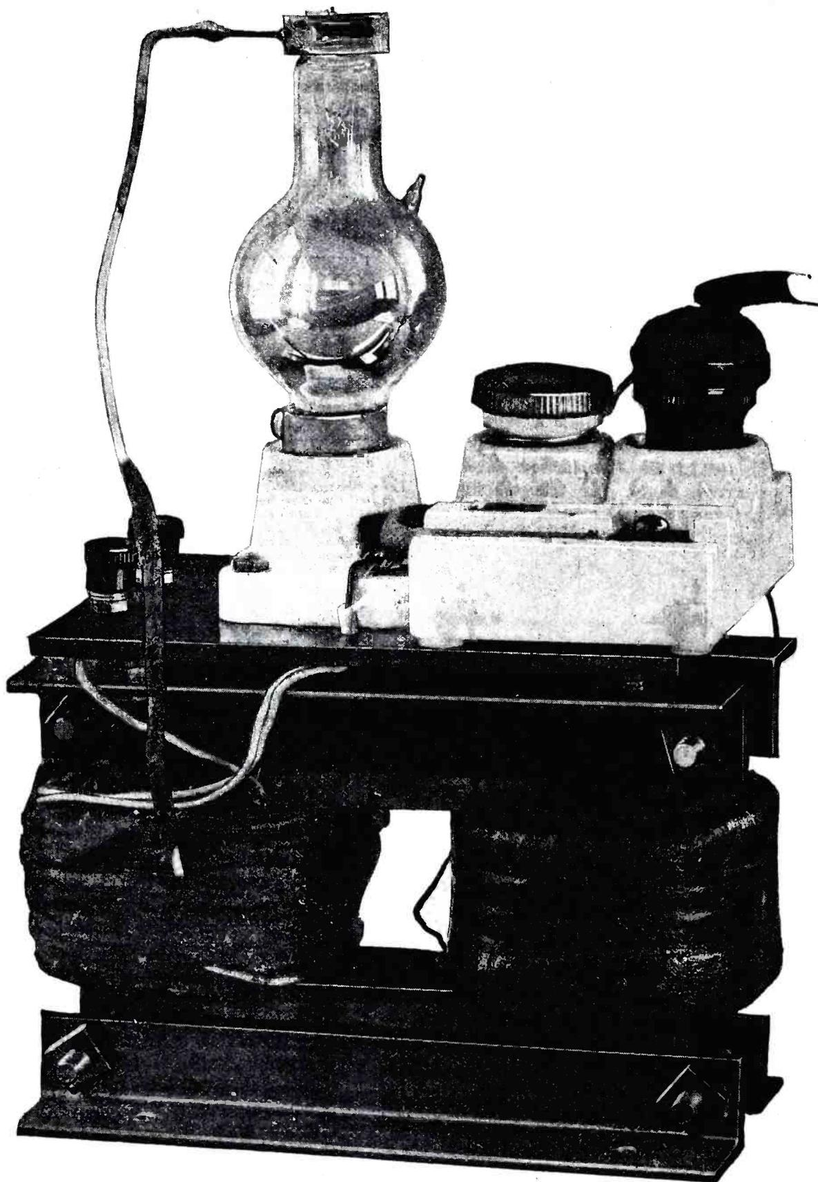
Fig. 4. How the made-up charger looks. A bakelite panel, situated above the transformer coil supports the output terminals, tungar tube, socket and input socket with fuse block.
