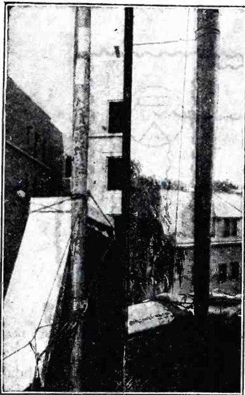
Fig. 1 (left hand photo), showing how one of the poles is held in place. This is at the slanting portion of the roof. Note the large amount of rope holding the pole. Fig. 2 (at right), showing how the pole which is at the cornice of the roof, looks. Note the guy wire coming down from the pole.
