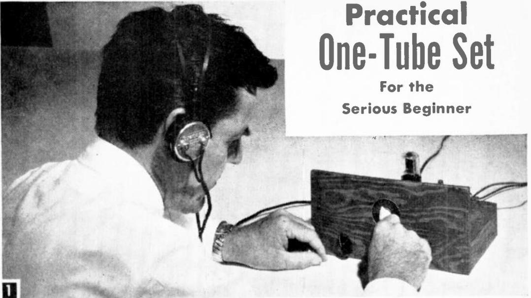
Unhampered by a tiny cabinet, the novice can easily put together this basic circuit in four stages, testing as he goes along to "see" how a radio works. Scrap wood panel and base afford room to rearrange or add parts.
