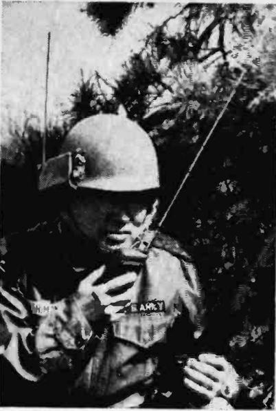
**HELMET HELLO.** A miniature radio receiver clipped to the side of a GI's helmet keeps him in constant touch with his company. Pocket transmitter enables soldier to hold two-way conversations to pass on vital information. Units are still being tested.
