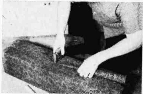
GRILLE CLOTH is used to cover column. Use staples until secured with upholstery tacks.
