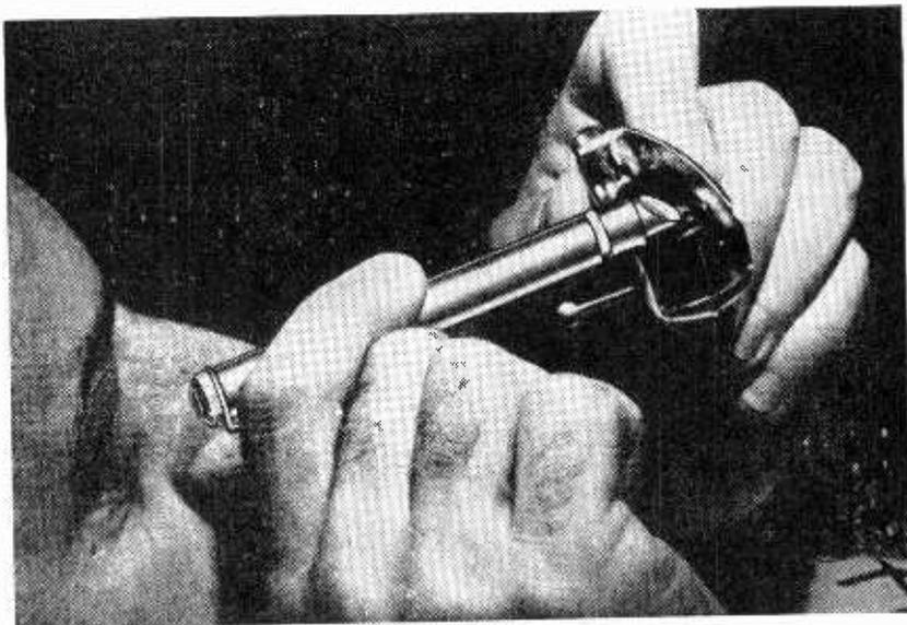
Seeing is believing—regular stylus inspection by means of a special stylus microscope will prevent disc damage due to unsuspected stylus wear.
