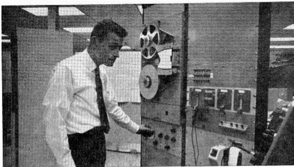
**Tape samples are tested from each production run. Tests, beyond normal listening are performed automatically by computers that rate the magnetic tape.**
