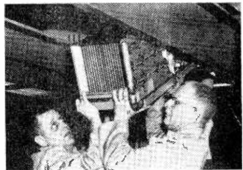
Solid-state air conditioner is being installed in existing air duct (top right). Complete unit is shown upper left with solid-state section located in middle. Diagram at left shows how room and outside air are mixed and cooled. Only fan blower and damper move.
