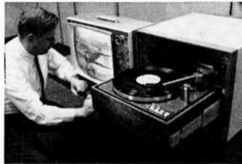
■ The *Videodisc* spinning above has more than sound in its grooves. It also stores video signals that are picked up by the stylus of a conventional record player and read out to a conventional television receiver. The unique part of the system, termed *Phonovid*, and developed by the Westinghouse Electric Corporation, is the link that joins record player to television receiver. The link is comprised of electronic circuits that make up what is known as a scan converter.
