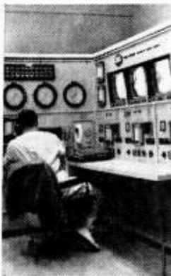
Television receiver screen on console is one of three that monitors activity in the three rooms or chambers of oxygen tank facility. Here, as in any form of technical communication, a picture is worth a thousand words, or in this case, it is worth valuable time that might be lost in diagnosing meter readings when a picture might reveal the nature of the situation within the oxygen chamber.
