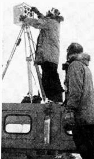
Distances across the vast and eerie Antarctic wastes were measured using electronic survey equipment. Protected by warm parka and beard, Boeing man adjusts the equipment which was mounted on snow vehicle to get it above the snow-whipped ground surface. As shown at the top, the men relaxed by conquering a mountain of snow near camp.
