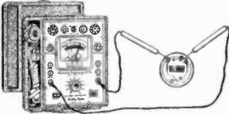
Avoid time consuming and embarrassing repair of appliances when the switch is suspect. Model 161 will indicate if the switch is okay, open, or has a faulty intermittent contact.
