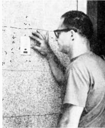
and cut-out the opening with a saber or keyhole saw. If your home is brick faced mount a waterproof electrical box on the brick and mount the remote in the box—most outdoor remote units have rubber seals for weather-proofing.
