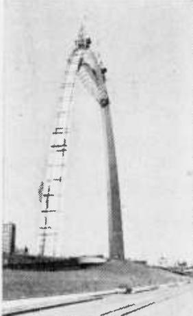
Highest U. S. monument, the 630-foot, \$30-million Gateway Arch rises majestically above St. Louis skyline, its welded joints 100 per cent inspected with the aid of nuclear energy emitted by a radioactive isotope. Its welded panels are designed to withstand winds of more than 150 miles an hour.
