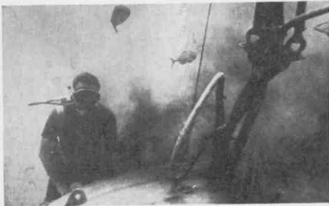
At 110 foot level, diver Ed Davies inspects cables connecting Sea Spider's underwater sphere to telemetering buoy at surface. The many inquisitive fish bring other, unwelcome visitors, dangerous sharks and toothy barracuda, to the experimental "inner space" anchorage.
