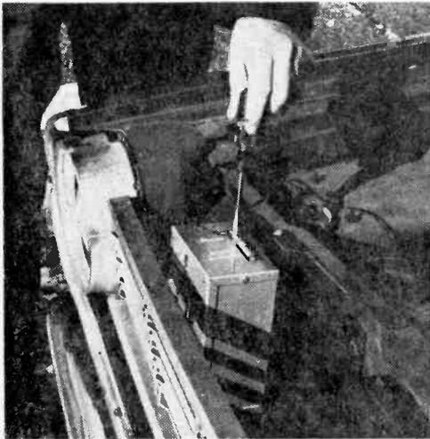
Once Auto Siren Sentry is attached to the body, leads to switches can be connected. Protect leads from accidental breakage and possible tampering through grill openings.
