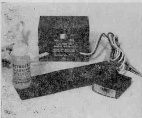
Basic metal marking kit contains transformer and cord, a clip and hand pad, oxidation chemical, and strips of the stencil material.
