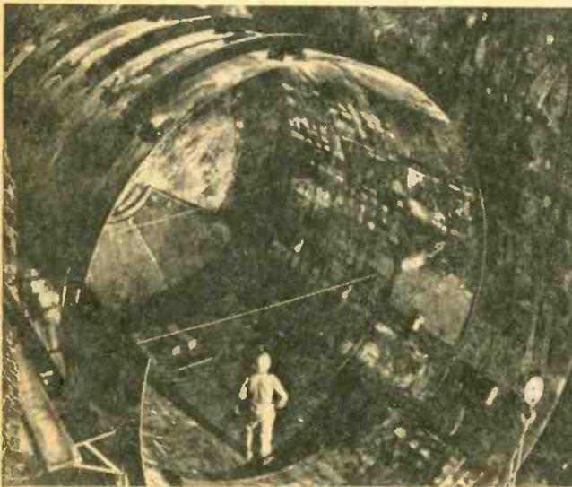
Miner's eye view of the Brookhaven Solar Neutrino Observatory at the bottom of the Homestake Gold Mine during construction. This tank, measuring 20 by 48 feet, holds over 100,000 gallons of perchloroethylene liquid which is used to detect the elusive solar neutrino. Nope, it can't detect gold.
