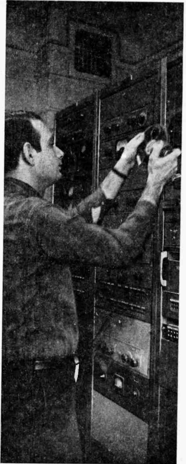
Getting ready to record High School of the Air program, station technician loads tape on recorder mounted in large rack panel.
