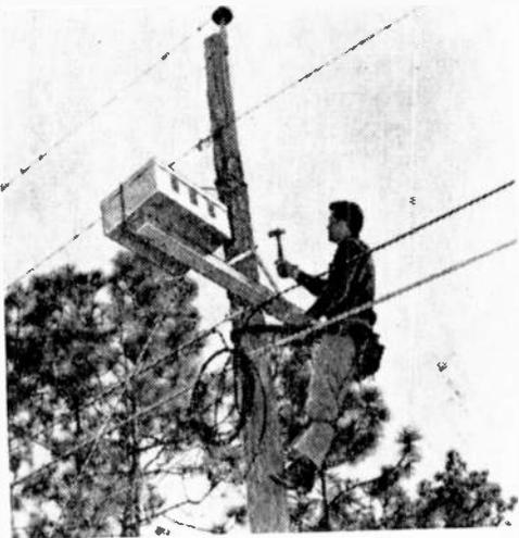
Signals from antennas feed trunk line which is main coax cable into town. Amplifiers are mounted on poles to boost distribution lines.
