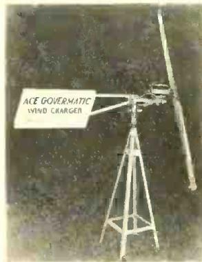
★ Charger for six volt batteries. Propeller automatically adjusts self to wind conditions—speed control safeguards generator from overload. Cut-out prevents overcharging. Ammeter shows rate of charge. Mounts atop barn or house. Special co-operative price of \$10 to purchasers of Crosley battery radios. Ace Products Corp., Cincinnati, Ohio.—**RADIO TODAY**
