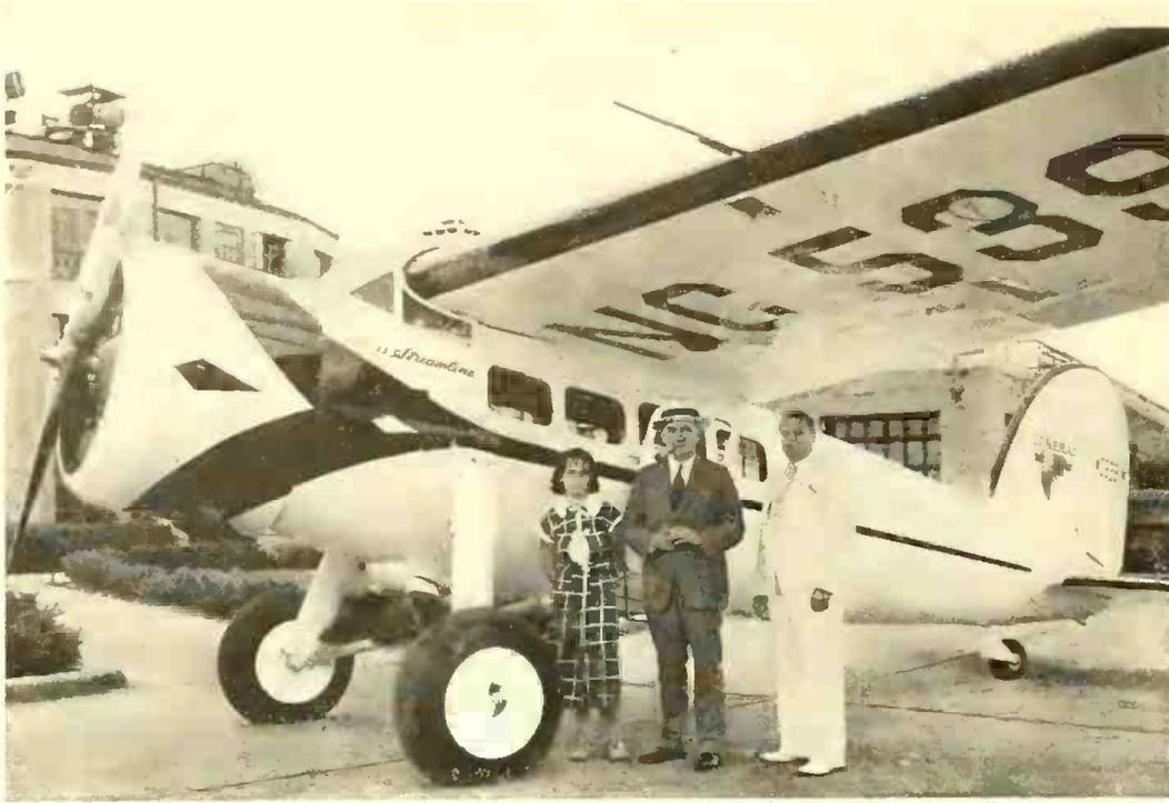
Guided only by a radio direction compass, tuned on broadcasting stations, this Lockheed Vega plane flew in one day around a 1,300-mile circle from New York to Cleveland and back to Washington.
