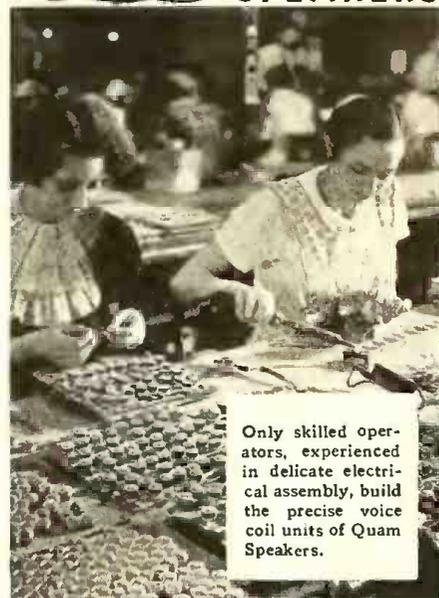
Only skilled operators, experienced in delicate electrical assembly, build the precise voice coil units of Quam Speakers.
