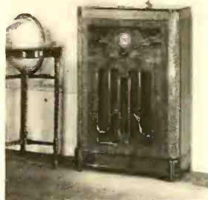
★ Three-band farm or summer cottage set for operation from storage battery. Seven tubes in superhet circuit—range, 540-1500, 1450-3500, 5600-18,000 kc. Full vision dial with dual-ratio vernier. Vibrator power unit—permo-dynamic speaker. Model 115. Stromberg-Carlson Telephone Mfg. Co., Rochester, N. Y.—RADIO TODAY
