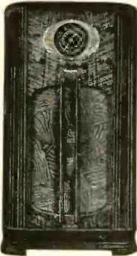
CONSOLE, WR-311. Standard, Foreign, and Police Bands, Spot-lite Tuning, Full-Automatic Volume Control, Continuously Variable Tone Control.
