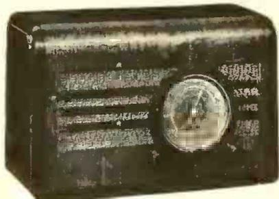
Model 87—dual band AC-DC superhet with 7 tubes including ballast. Range—550-1600, 5500-15,500 kc. 2-gang tuning condenser— $4\frac{1}{2}$ -inch dial with planetary drive. Six-inch dynamic speaker. Size 10 x 16 x  $6\frac{3}{4}$  inches—walnut cabinet. List \$29.95.
