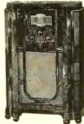
Four-band hi-fi console. Tri-focal tuning with 6E5 cathode-ray tuning indicator. Edge-lighted selectorlite dial—micrometer sub-dial. Metal tubes—beam audio output of 30 watts. Acoustical labyrinth and carpinchoe speaker. Model 160-L—list \$275.
