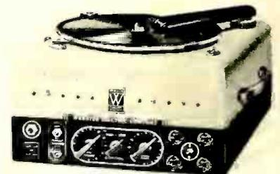
★ 6-volt and 110 AC amplifier for mobile use. Has phono and microphone inputs which can be mixed. Four speaker receptacles with change-over switch to match speaker load. Crystal pick-up. Modernistically styled base and hood. Webster Electric Co., Racine, Wis.—SELLING SOUND—see also advt. p. 2.
