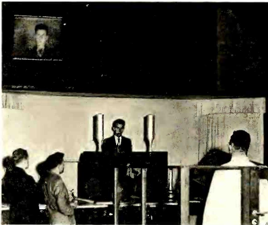
At the Berlin Radio Show, this cathode-ray outfit re-projected an enlarged picture of the speaker, onto a screen behind him. Scanning was accomplished by a flying-spot of ultra-violet, cathode-ray controlled.
