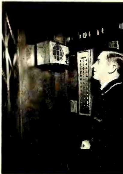
This Bogen wireless interphone provides communication between the elevators and gives better service in the absence of a starter. Unit installed by Thurow Radio of Jacksonville, Fla., attracted wide attention and pleased the tenants of the building.
