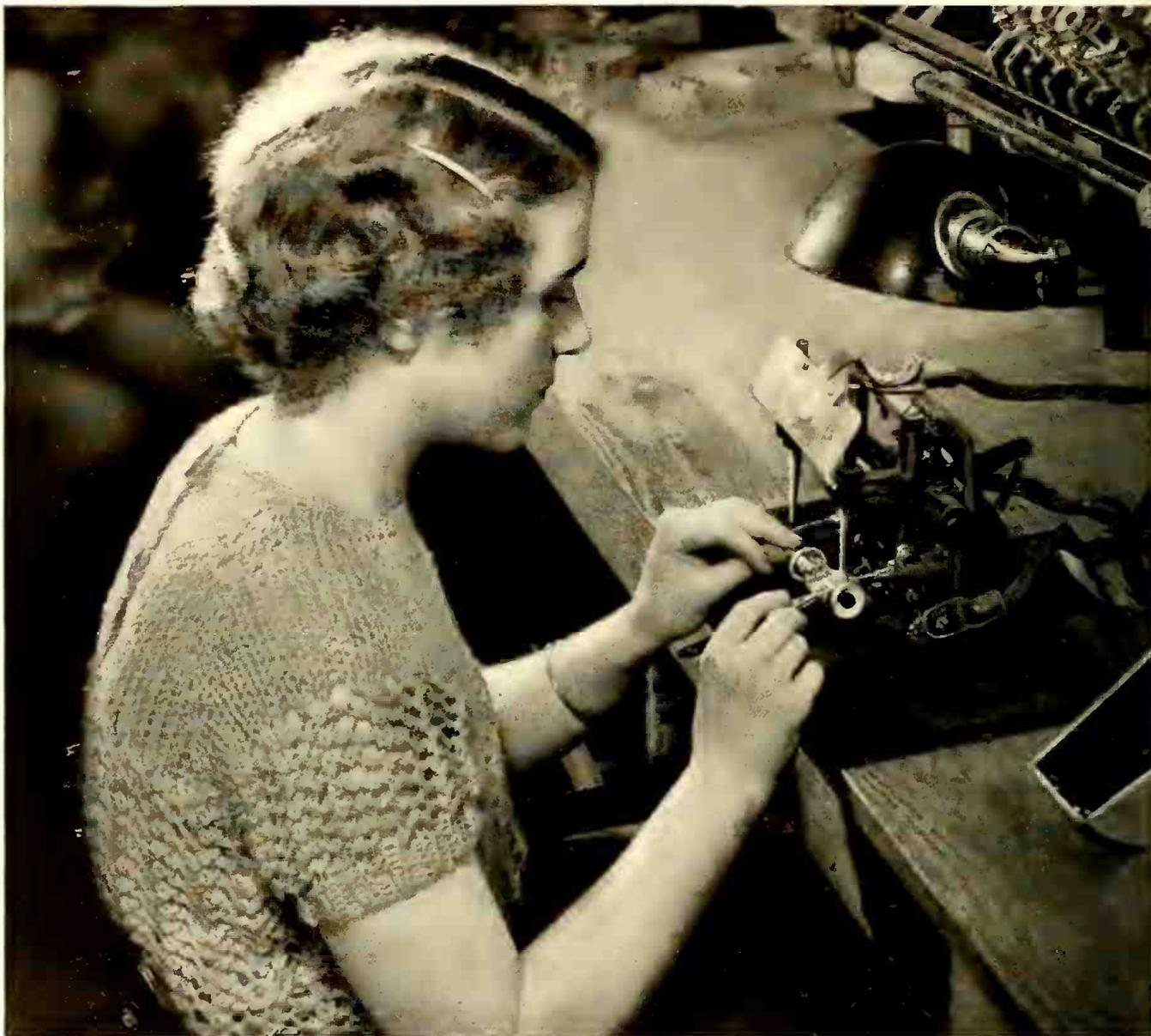
ONE of the most delicate processes in Sylvania tube manufacture is "mount assembly"—a job that demands exceptional precision and skill. For each tube part must be accurately spaced in relation to other elements . . . and carefully welded in place.
