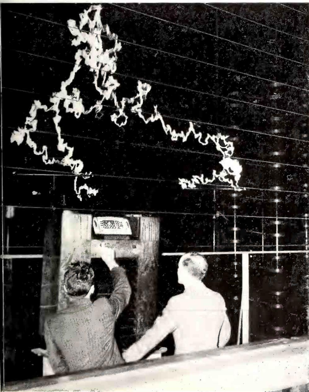
FM's ability to bring in noise-free reception despite powerful manmade or natural static, is shown in this test in the GE Building at NY World's Fair. Interference source—million-volt arc; reception—undisturbed!
