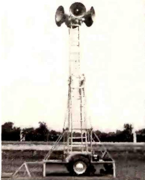
The unique mobile speaker-tower shown above and at right uses extension ladders for the tower, and 6 University Labs. LH projectors. Owner is Jack Kyler, Evansville, Ind.
