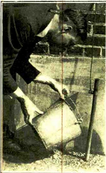
**RAYMOND B. WALES**, of 911 23rd St., Washington, D. C., shows the world how to make a good outdoor ground. To make sure that the earth surrounding the pipe is always a conductor of electricity, a bucketful of a copper sulphate solution, commonly called bluestone, and which is cheap, should be poured around the pipe. The solution prevents corrosion and is highly conductive. An iron pipe is used for ground connection.
