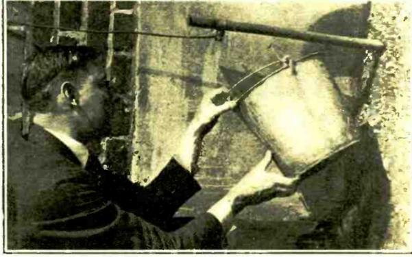
**RAYMOND B. WALES**, of 911 23rd St., Washington, D. C., shows the world how to make a good outdoor ground. To make sure that the earth surrounding the pipe is always a conductor of electricity, a bucketful of a copper sulphate solution, commonly called bluestone, and which is cheap, should be poured around the pipe. The solution prevents corrosion and is highly conductive. An iron pipe is used for ground connection.
