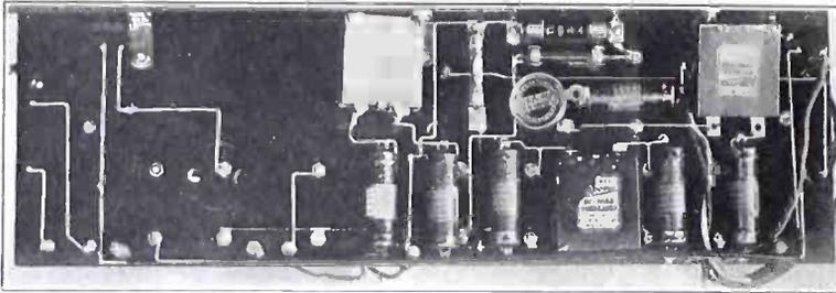
**THE BOTTOM VIEW.** Note how the arrangement of parts simplifies the wiring. The 50,000-ohm resistor (grid circuit of tube No. 5) is the one at right, directly above the central bypass condenser. (Fig. 6.)
