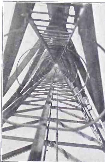
A BIRDSEYE VIEW up one of the 820-foot steel masts of the new radio station at Hillmorton, near Rugby, England. This is the first step of an imperial chain of radio transmitting stations, which will send commercial radio messages around the world. The complete station covers an area of over 900 acres. The power output of the station is 100 kilowatts. The signals are transmitted on a wavelength of 6,000 meters. (Acme.)
