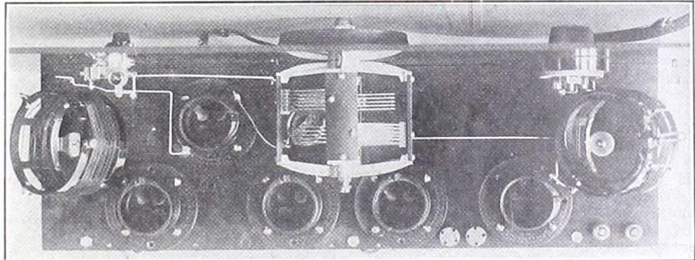
THE TOP VIEW (Fig. 5). The coil L1 L2 is at left, while L3 L4 is at right. The RF socket is at left, the detector socket between condenser C1 and coil L3 L4 (foreground). The audio runs in the opposite direction—first AF at right rear, then second and third AF in the same row. The phone tip jacks are to the left of the third AF tube.
