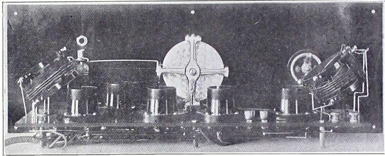
THE REAR VIEW (Fig. 4) shows the coils mounted at an angle of about 57 degrees, simply as an extra safeguard against stray coupling. The aerial and ground posts are at right. The two cup-like objects a few inches to the left of these posts are the phone tip jacks. The speaker cord tips are inserted here. The sockets are, left to right: first AF, detector, second AF, third AF and RF, i.e., as designated in Fig. 1, they are 3, 2, 4, 5 and 1.
