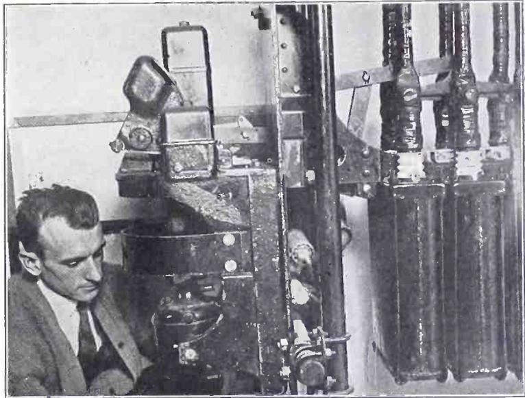
ONE of the motor-operated oil switches of WJZ's super-power station is at left. Although in a separate building, this, like all other switches, is operated from the control board in the operator's room. Note the huge condensers at right. (Kadel & Herbert.)
