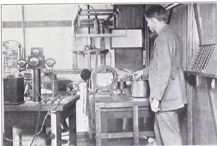
BETTER results from your radio receiver will result from experiments now being carried on by the U. S. Bureau of Standards in determining power losses in electrical insulating materials at radio frequencies. M. S. Strock of the radio laboratory, is shown engaged in making some of the tests. (Underwood & Underwood.)
