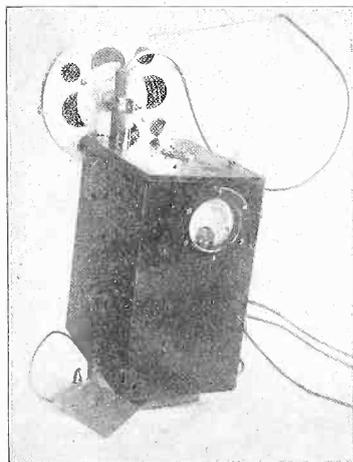
THE EMERGENCY transmitter which apparently was not given an opportunity to prove its worth. It is entirely waterproof. Everything from the key, which is under the little rubber diaphragm on top, to the batteries was inside. The ground plate and antenna reel were attached to the outside of the box. A small code chart is on the side, to the left. This outfit was identical as the one on the America, the Pride of Detroit, and the Royal Windsor.
