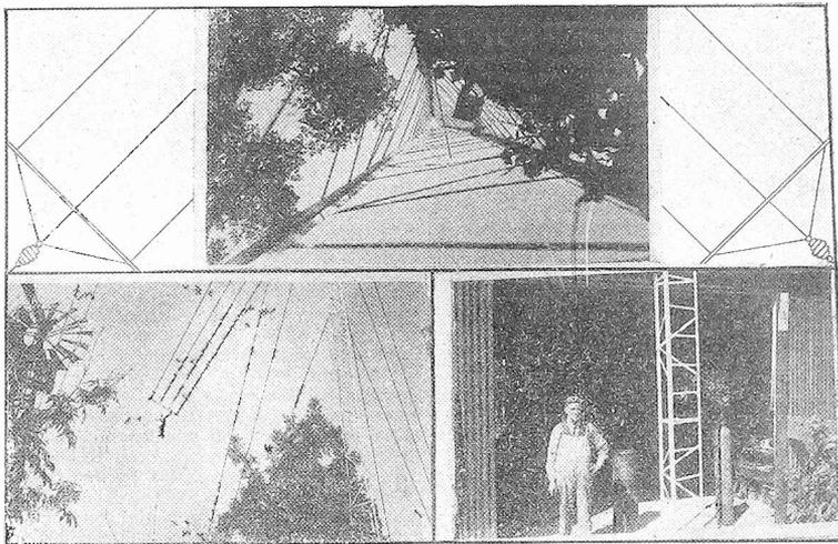
Upper—Looking up through the lattice of a welded aerial. This construction will survive high winds.
