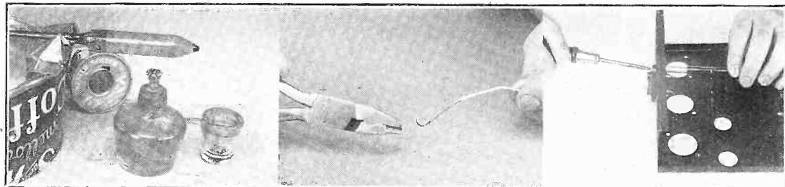
Can't read the brand of coffee on the label, but can is upside down, tin cover cut to remove coffee (just as important as anything else), and elevated resting place provided for soldering iron that needs alcohol lamp or pepper pot soup to become useful. Special pliers make neat lug end on wire. Socket wrench spares fingers for tightening in cramped places.
