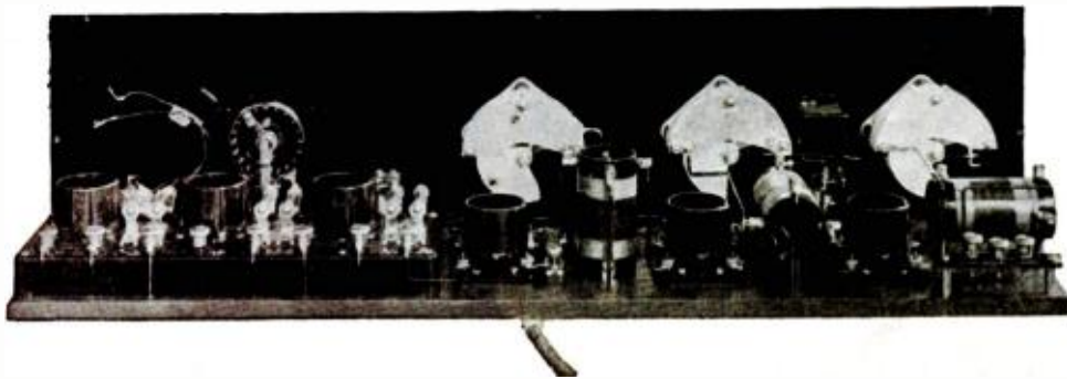
A view from the rear showing the instruments mounted on the panel and base-board.
