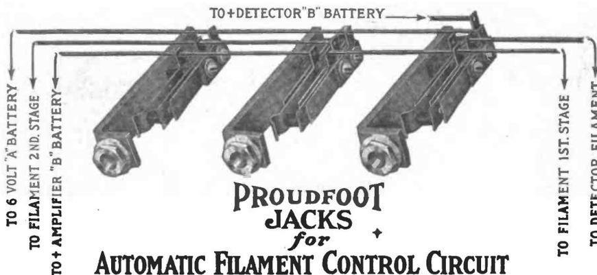
PROUDFOOT JACKS for AUTOMATIC FILAMENT CONTROL CIRCUIT DETECTOR & TWO STAGE
