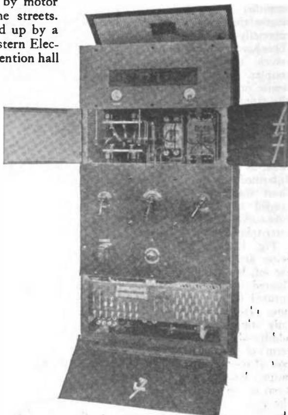
Radio Corporation 100-watt Radiophone Transmitter Used in Test
