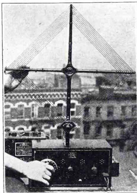
Fig. 1. Monotrol Set with Loop Aerial
