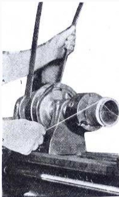
Fig. 2. Correct Position for Holding Wire
