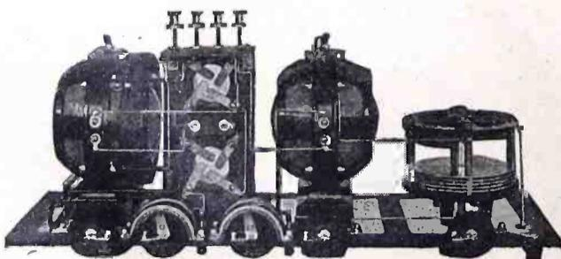
The Grebe "13" receiver is a short wave development, 80 to 300 meters, of the circuit employed in the "CR-12"; it employs two specially designed variometers with "split" windings and a stabilizer for control-
