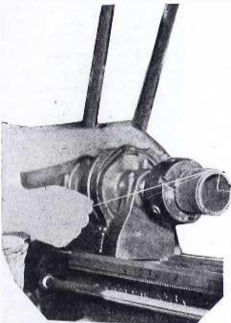
Fig. 1. How to Mount Tubing in Lathe
