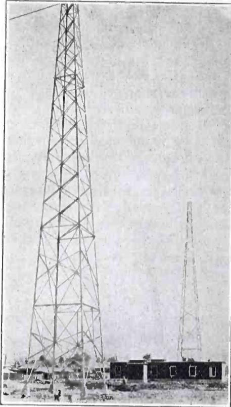
*Antennae towers, 150 ft. high, for the new General Electric Company broadcasting Station at Oakland, California*
